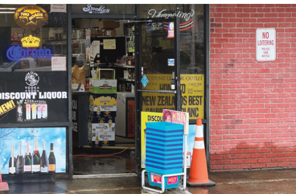
As a result of the severe weather rain storm on July 16th, Discount Liquors at 20 Potuccos Ring Rd. suffered interior water damage when their parking lot got flooded. Several streets and small bridges were compromised in several parts of town as a result of this storm and the volume of water it produced.
