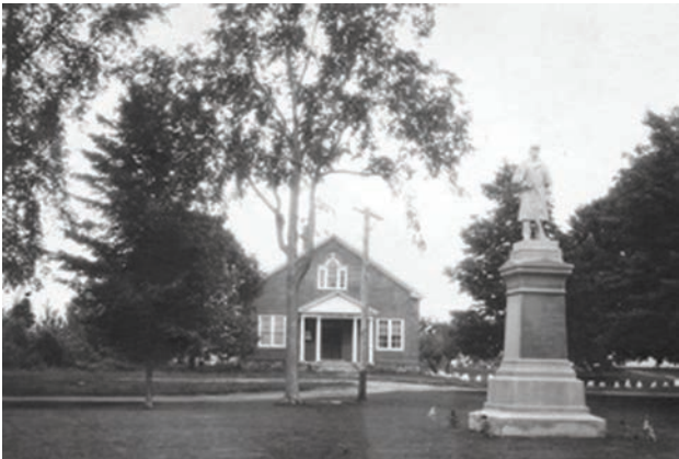
The 1923 structure that was included in the new construction/renovations from 1989-1991.
