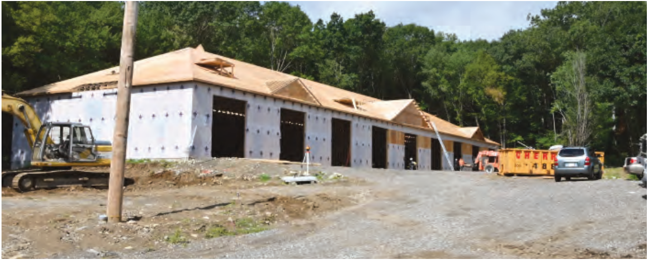
A new commercial building that can be subdivided for various commercial businesses is being constructed at 239 Wolcott Road. Research indicated there is a need for this type of building for businesses to utilize to store materials or vehicles or serve as office space to run businesses out of.
