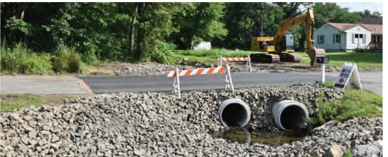
The Wolcott Public Works Department has been making repairs and upgrades at various locations in town that tend to flood during heavy rain downpours. This location on Longmeadow Drive near Wolcott Road had two large concrete pipes installed to handle such rain events and hopefully reduce or eliminate future flooding issues to local businesses.
