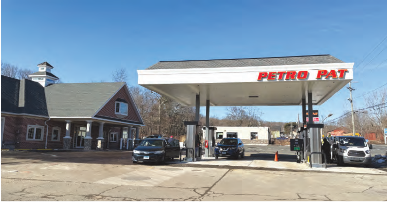
The new Petro Pat gas station and convenience store located at 685 Wolcott Road is officially open for business. The construction of a new building and state of the art gas pumps with a canopy has finally been completed. An official grand opening is being planned in the spring. Photography by Picard
