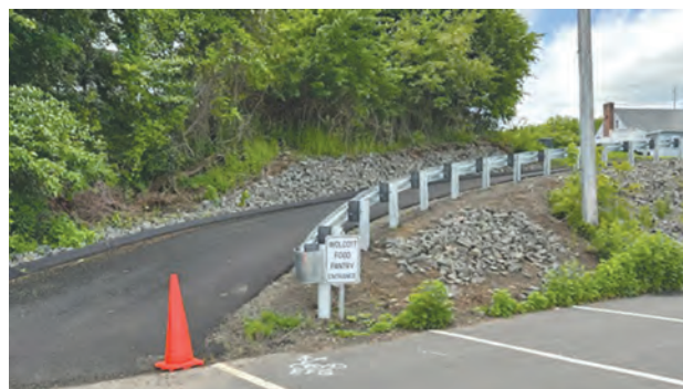
The town is adding some finishing touches to the new access road leading to our distribution canopy. The road has eliminated a big traffic issue on Woodtick Rd. and we are relieved we are able to utilize it during food distributions.
